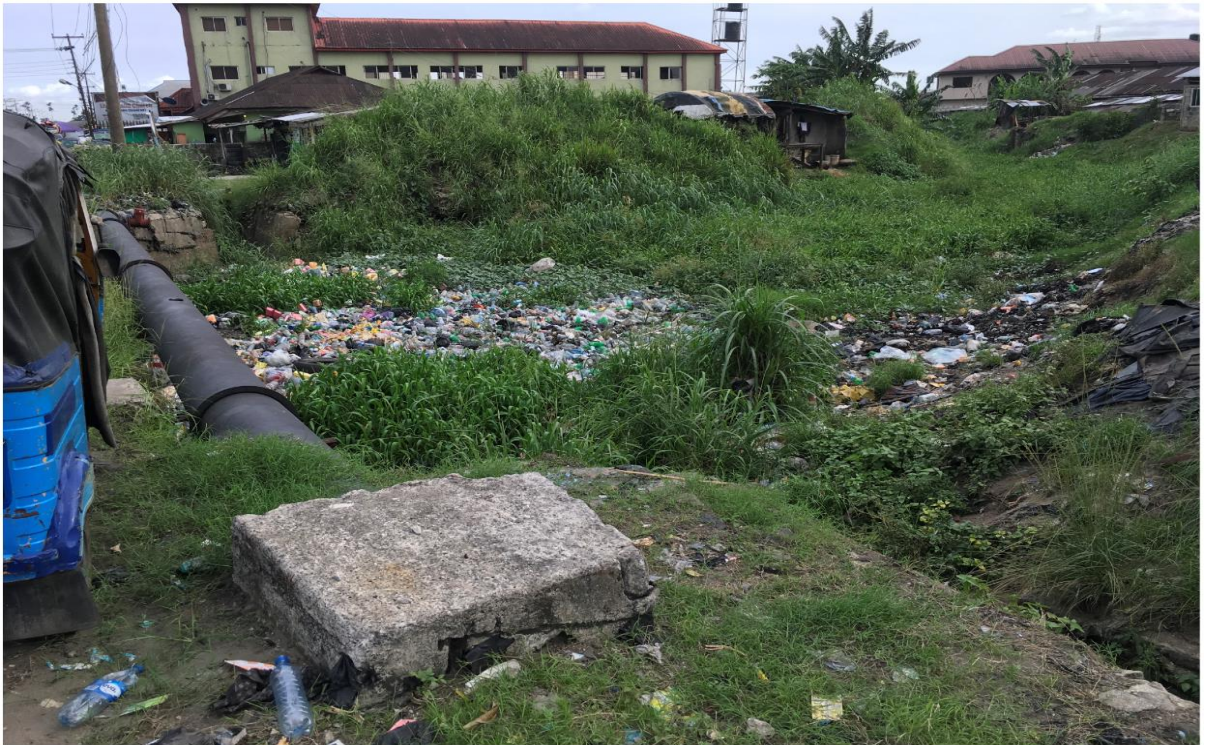
Figure 4: BLOCK WATERWAY ON UGBOGBOROCREEK ACROSS DECO ROAD, WARRI
