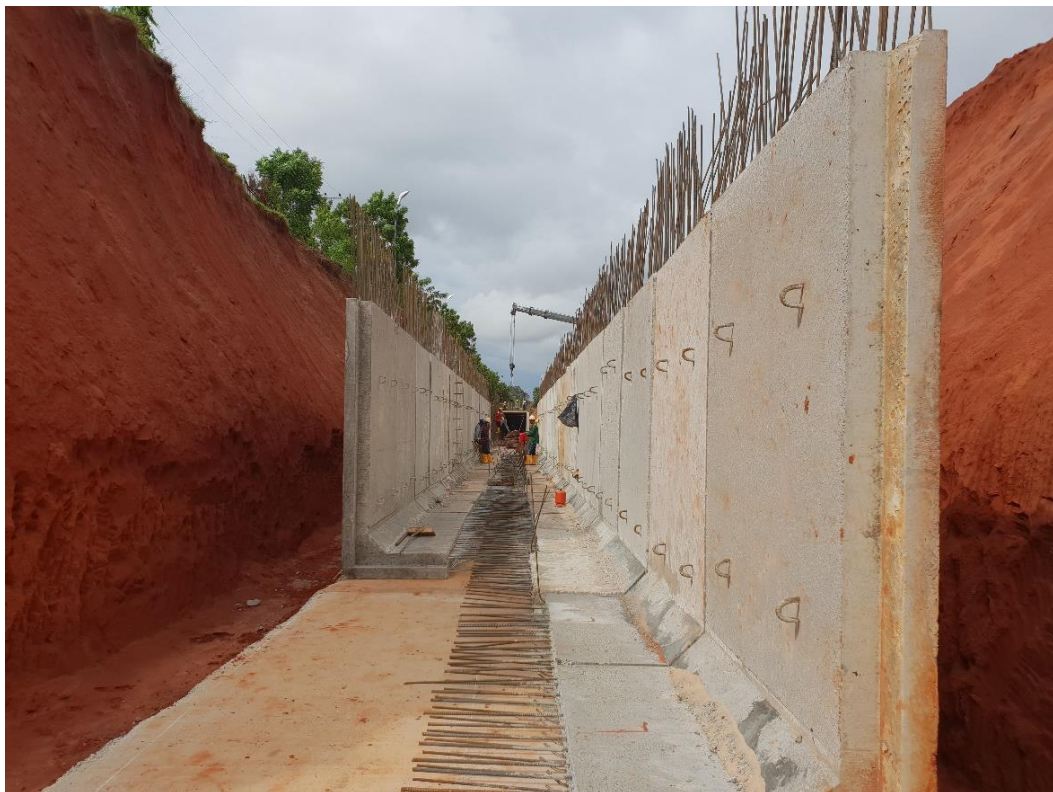
Figure 15: L-Shaped Precast Stormwater Sewer Channel under construction
