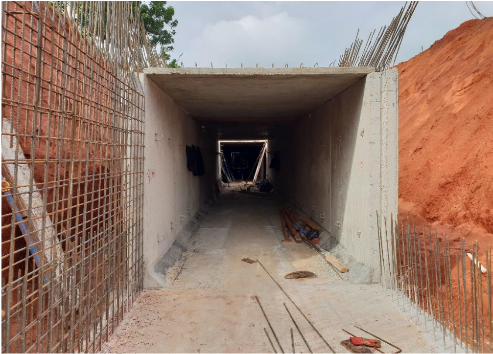
Figure 16: Completed Rectangular Precast Stormwater Sewer Channel
